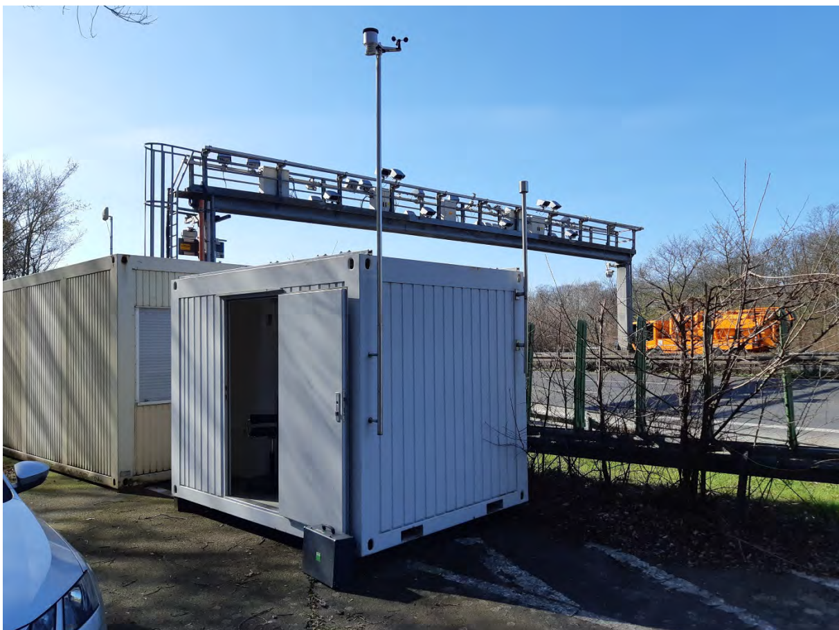
Figure 7: Measuring station used for conducting the field test
