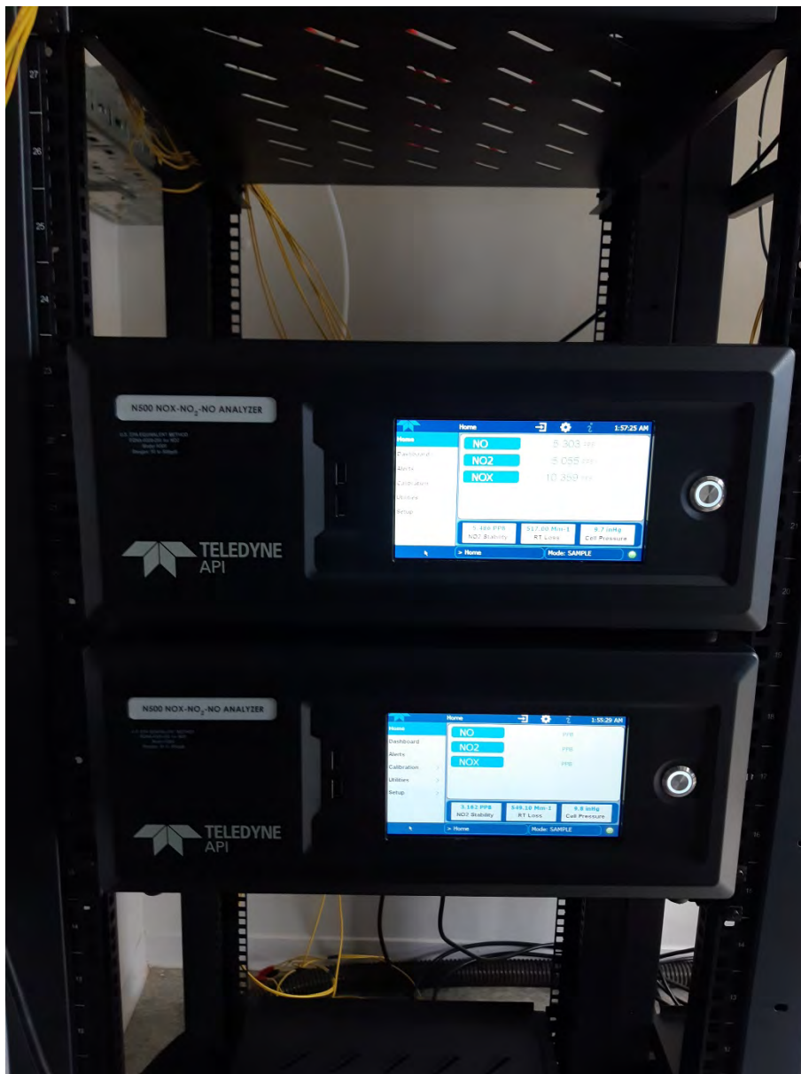
Figure 8: N500 in the measuring station during the field test
