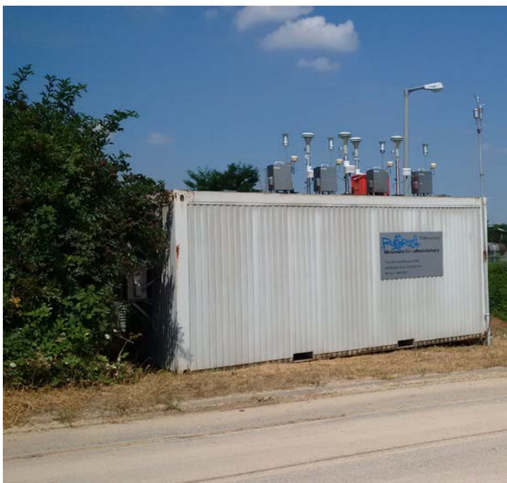
Figure 5: MP101M measuring systems on the measuring station (bulk handling)
