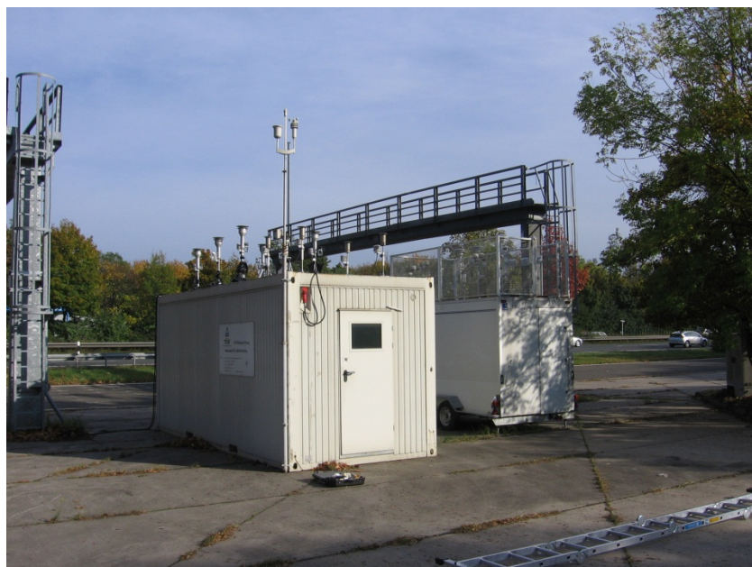
Figure 19: Field test site Bornheim, motorway parking lot
