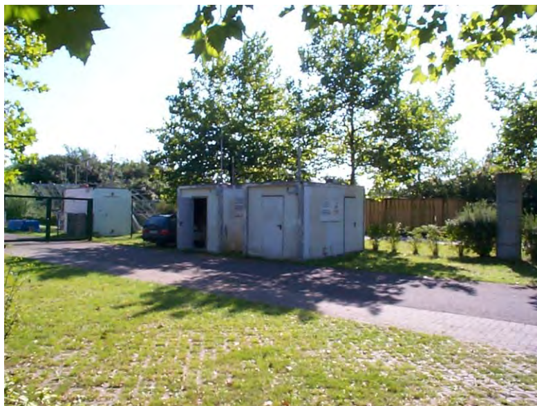
Figure 19: Field test site „Cologne, parking lot“
