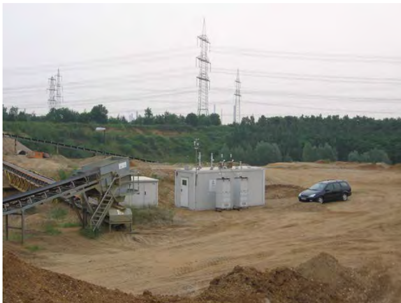
Figure 29: Field test site Bruehl
