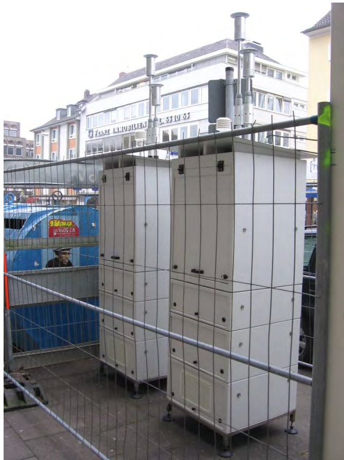
Figure 11: Outdoor measurement racks at the field test site in Bonn, Belderberg
