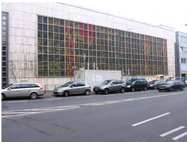
Figure 27: Field test site Bonn, Belderberg
